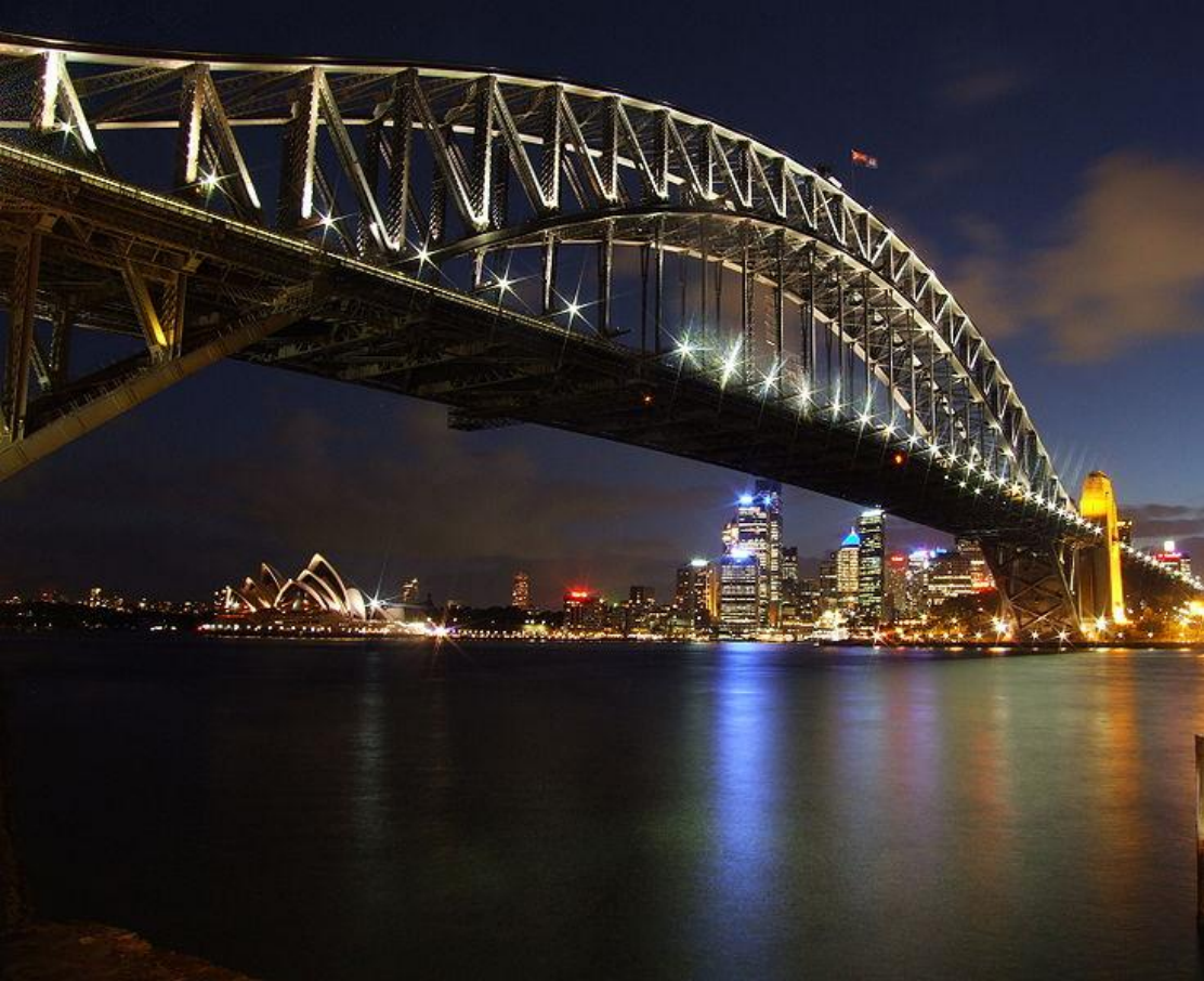
THE HARBOUR BRIDGE, SYDNEY
